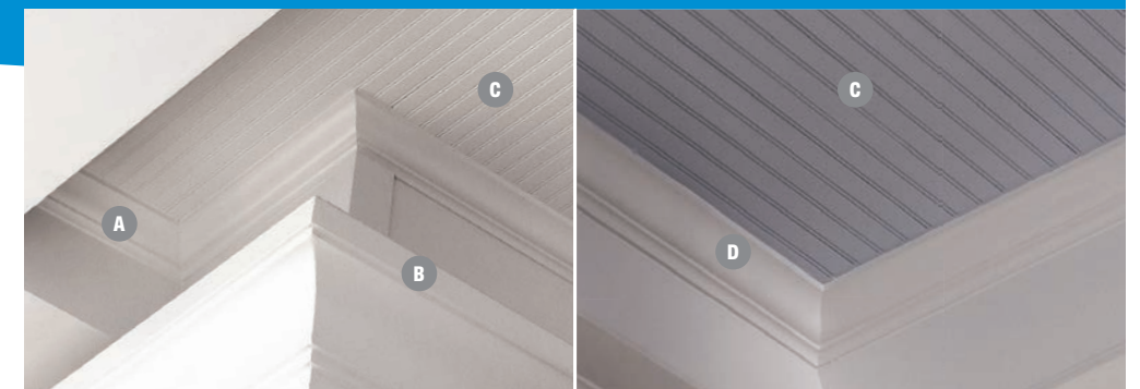
A Crown B Bed Mould C Beaded Planking D Scotia/Cove
